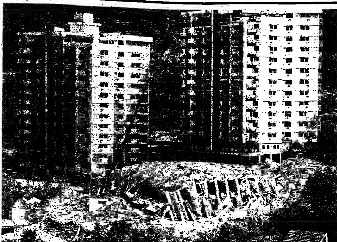
ONLY RUBBLE LEFT — A 12-story apartment block outside Kuala Lumpur collapsed after it was hit by a landslide, killing at least one person. About 50 people were believed trapped in the ruins. Nearby apartment blocks have been evacuated as a precaution. A consortium signed a contract last month to build twin 85-story office towers in the city that would be among world's tallest.
